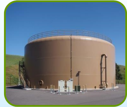
Appian Tank, Union City Retrofitted for earthquakes
